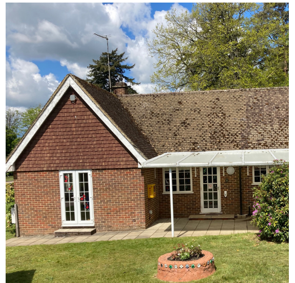
Little Court building where the new facility will be housed.
